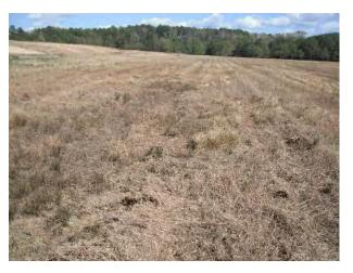
**LF4-004:** Four areas of minor subsidence were observed south of the centrally located drainage ditch. These areas appear to be areas that hold water during the wet seasons. The areas will be repaired during Phase II of the Industrial Landfill closure.
