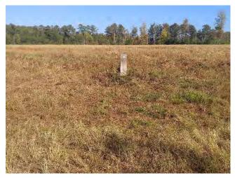
LF3: The vegetation across the cap surface was in good condition at the time of the inspection. Two no digging signs were observed to be missing but replaced at the time of the inspection.
