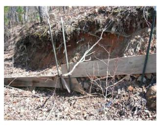
The t-posts located behind the wooden board helps to keep the board in place and helps limit erosion.
